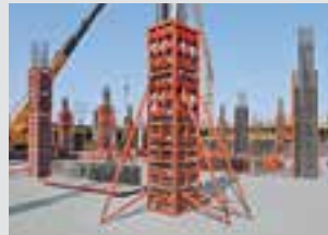
Column Formwork
