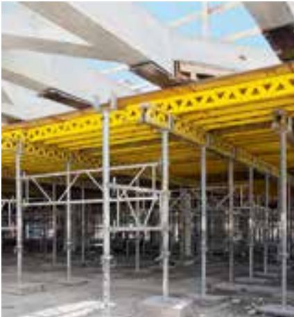
The MULTIFLEX Slab Formwork - configured with GT 24 Formwork Girders – supports the formwork for a "network" of architectural concrete balconies which later supports a prefabricated slab.
