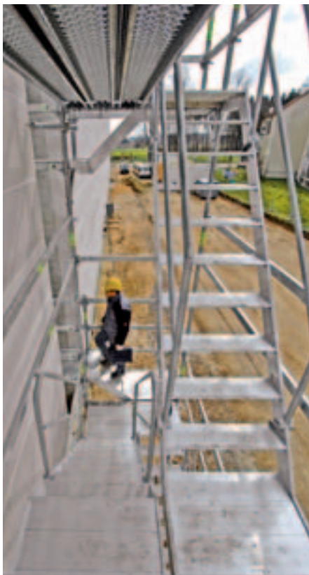
The lateral height adjustments leave the landings free for climbing up or down.
