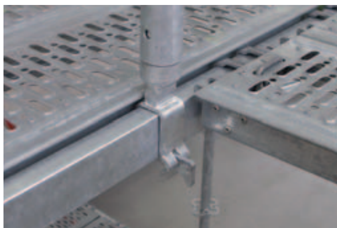
Standard-to-ledger connection.
