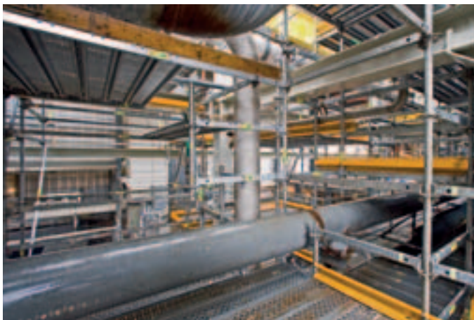
Guardrails and toe boards can be adapted to suit site conditions.
