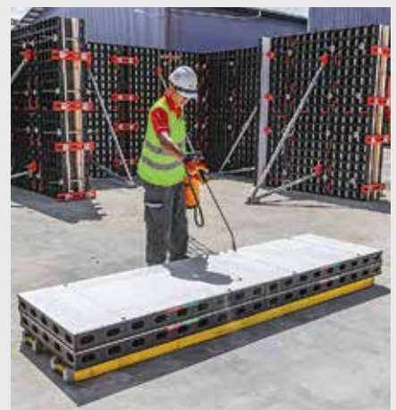
The release agent PERI Plasto Clean can be applied easily using the release agent pressure sprayer.
