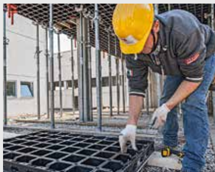
4. Screwing on the new formlining
