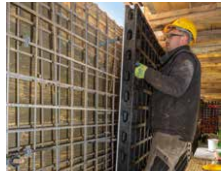
The lightweight DUO formwork elements were perfectly suited to building redevelopment.
