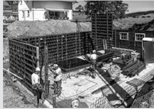
Wall Formwork
