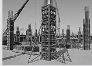
Column Formwork
